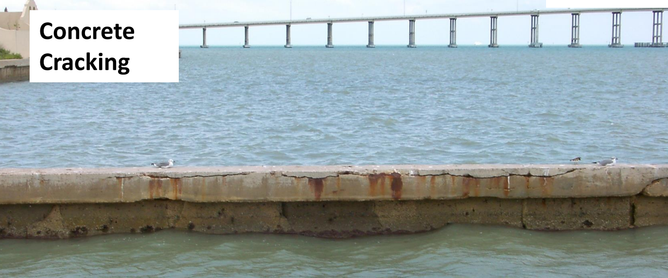
Concrete Spalling
