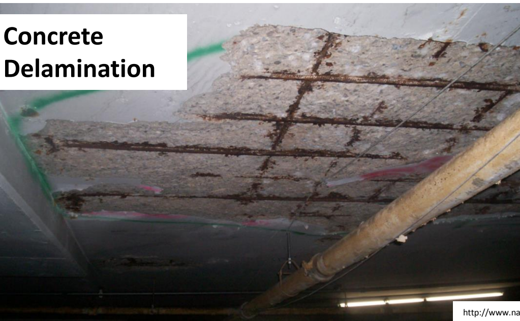
Concrete Structural Capacity Impacted
